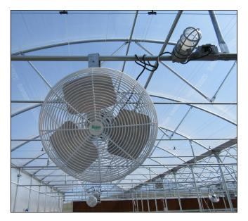
**Fan location** - The HAF fans should be located 2 to 3 feet above the plants and aligned parallel to the side-walls of the greenhouse so that the air is circulated around the house in a rotational pattern.
