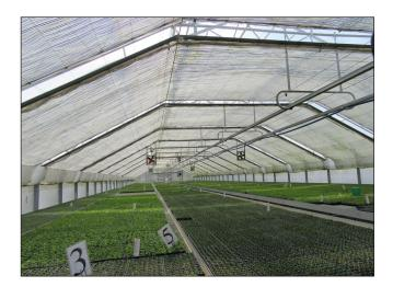
**Installation details** - Make sure that the blanket fits the greenhouse walls tightly to reduce heat loss above the blanket. Heating or water lines should be located below the blanket or be well insulated to reduce heat loss.
