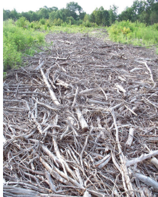
Figure 3. Logging residues utilized to stabilize a skid trail.
