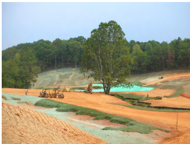
Figure 4. Hydroseeding at Ballyhack.
