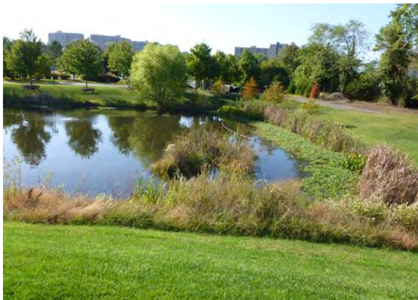
Figure 14. After: Storm water management pond using bubblers and floating wetlands to control nutrient enrichment and aquatic plant growth.
