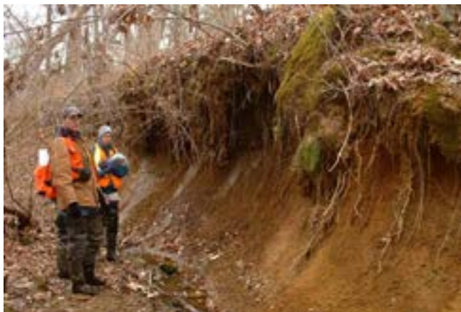
Figure 1. Eroded gully due to urban runoff. (Image courtesy of Erik Michelsen, Anne Arundel County Department of Public Works. Used with permission.)
