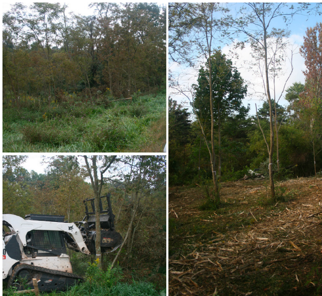
Figure 5. Mulching is a good way to clean up a site quickly and with minimum disturbance (as compared with bulldozing), but the benefits must be weighed against generally greater expense. (Photos by John Fike.)
