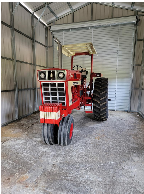
Figure 1. Repurposing a concrete slab from a corn crib into dry storage with a pre-engineered building.
