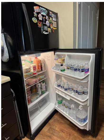
Figure 2: A refrigerator door with shelves filled with plastic water bottles that will act as a temperature stabilizer (Chojnacky et al., 2009). (Source: Ellen Gabriel)
