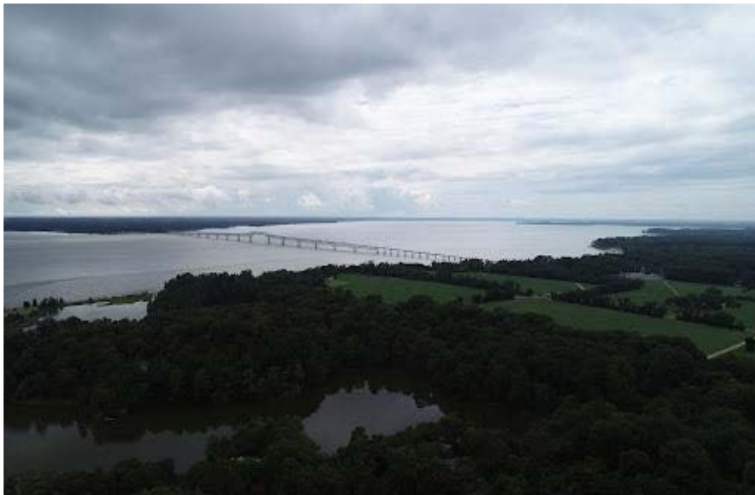
Robert O. Norris Jr. Bridge. (Trent Jones, Virginia Cooperative Extension)
