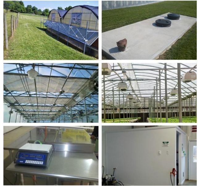
Figure 2. Site and infrastructure characteristics to consider, including site layout and adjacent land use (top left); well water system (top right); structural framing, supports, and lighting (middle images); packing areas (bottom left); and restroom facilities (bottom right). (Amber Vallotton, Virginia Cooperative Extension)
