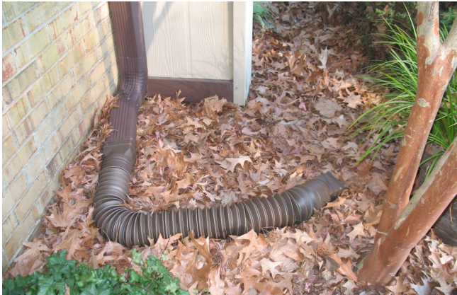
Figure 2. Example of a downspout with a flexible extension pipe. Direct the runoff 10 feet away from the foundation and into the landscape. Photo by Mary Ann Kincaid, Virginia Beach Master Gardener Water Steward.
